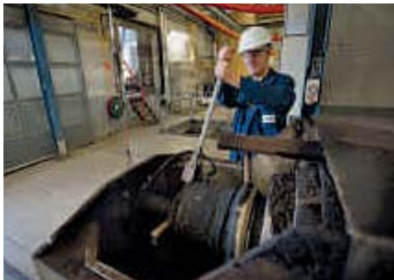
At Joure in the Netherlands, Veolia Energy — Dalkia helped coffee roasters Douwe Egberts Master Blenders convert to biomass. This transformation reduced the plant's carbon footprint by 14,000 metric tons of CO 2 a year.
