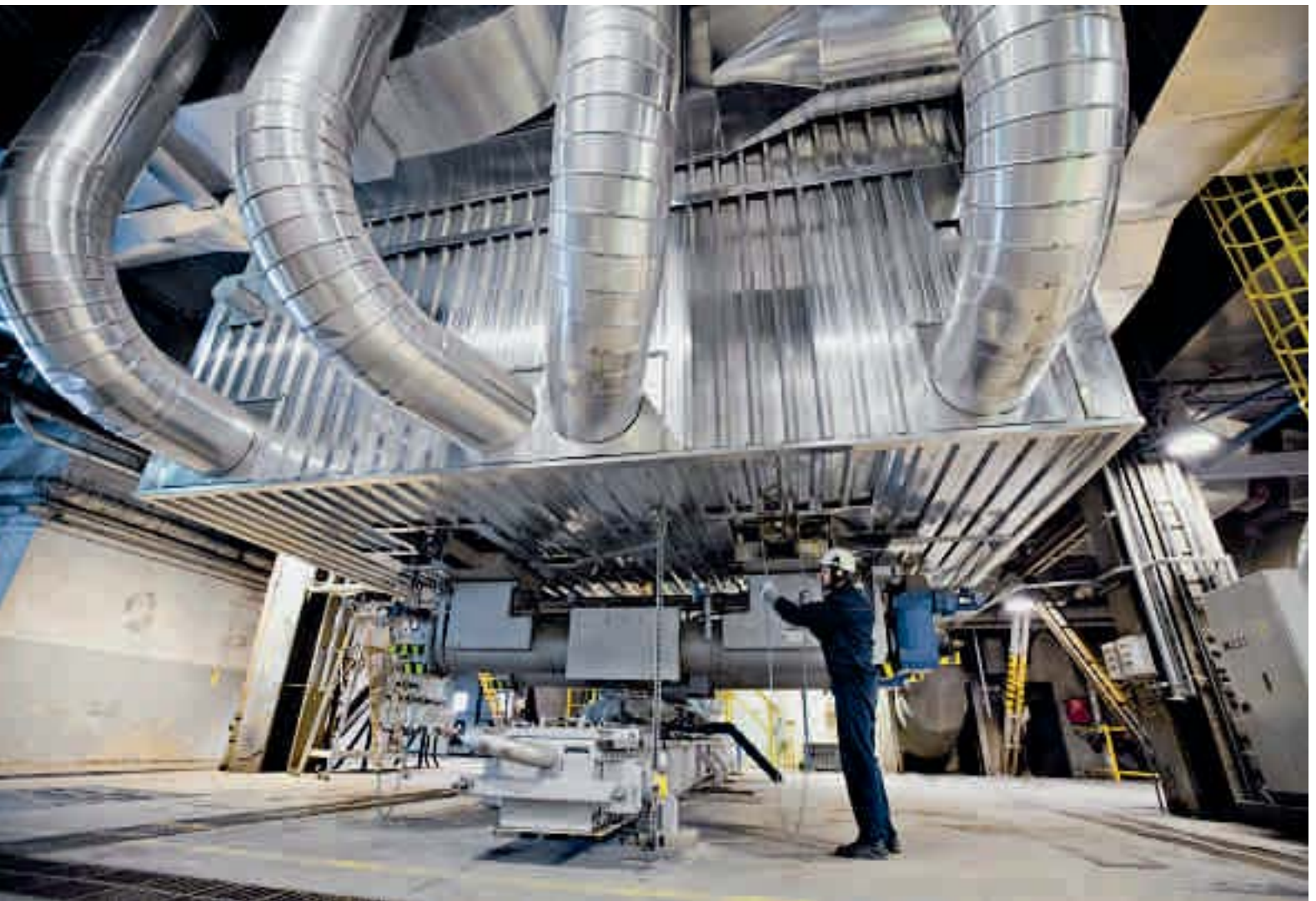
In Poznań (Poland), a 100% biomass-fired boiler now supplies the city's district heating network.
